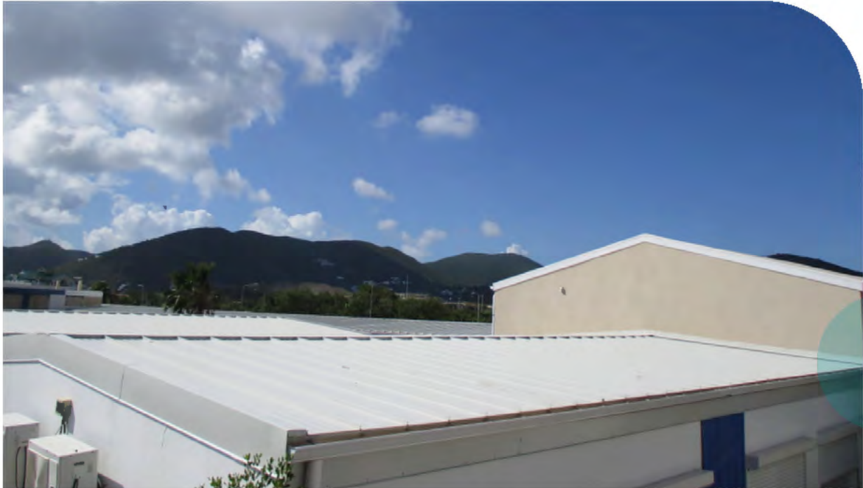
Nineteen school structures have been repaired and structurally refitted, creating a safer environment for students and staff post-Hurricane Irma, and strengthening resilience to future hurricanes. (Photo credit: NRPB)
