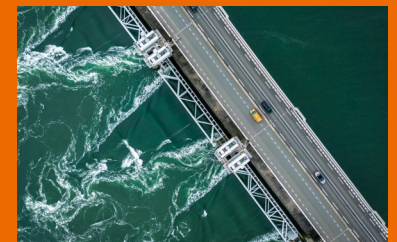
Declared one of the Seven Wonders of the Modern World by the American Society of Civil Engineers, the Delta Works are emblematic to future-oriented thinking and climate change resilience.
