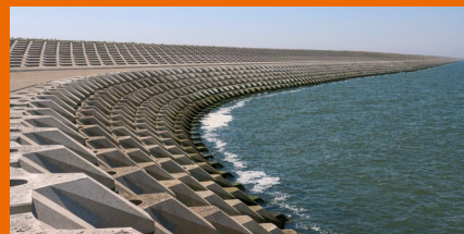
Financed as an eligible expenditure with the Dutch Green Bond, these Level-Blocs save up to 56% of CO 2 emissions in construction.
