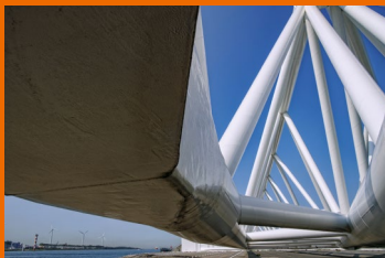
The Maeslantkering is a storm surge barrier and part of the Delta Works. This system can automatically close when it detects a flood, making it one of the largest moving structures on Earth.
