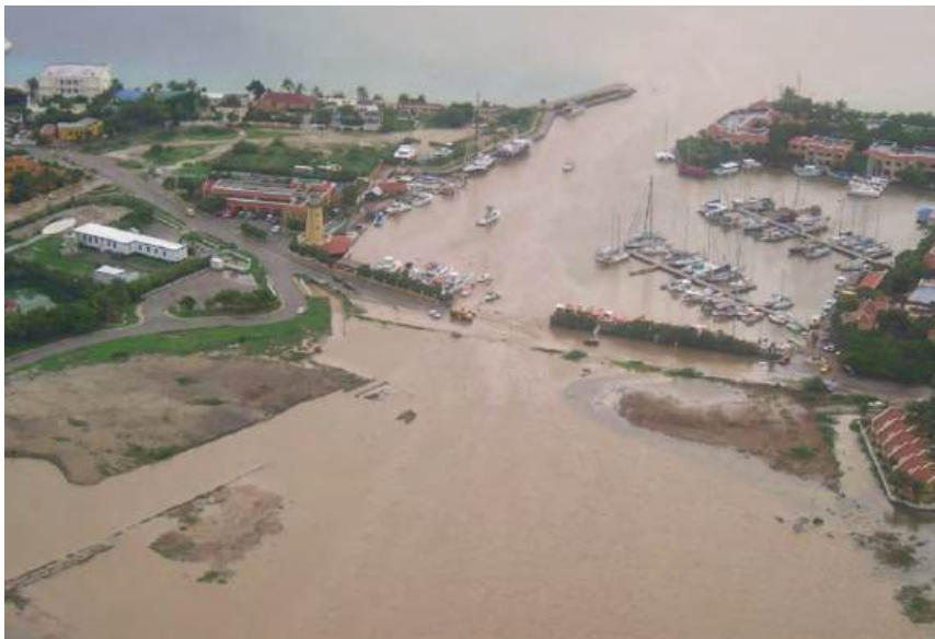
Figure 4.3 Sediments entering the sea from Saliñas di Vlijt after heavy rainfall. Photo by: © Directie R&O
