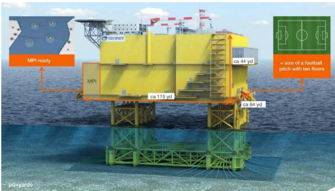
Figure 6.18: Standard 2GW HVDC platform (ref. 44).
