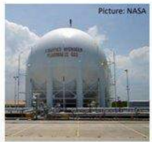
Picture: NASA NASA, 3800 m 3 , 270 t Boil-off ~12% H 2
