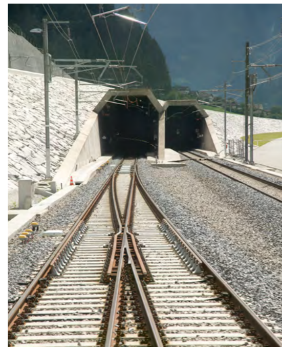
The north portal of the Gotthard Base Tunnel in Erstfeld.
