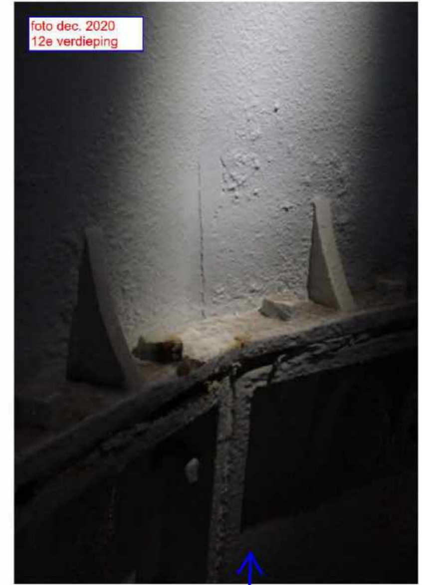
Verticale scheur in wand
