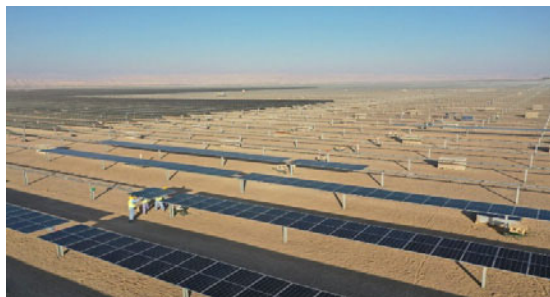
Workers installing one of 1.4 million solar panels that make up the Ibri II 500-megawatt solar photovoltaic independent solar power plant, the largest utility-scale solar park in Oman. Photo © AIIB 2021
