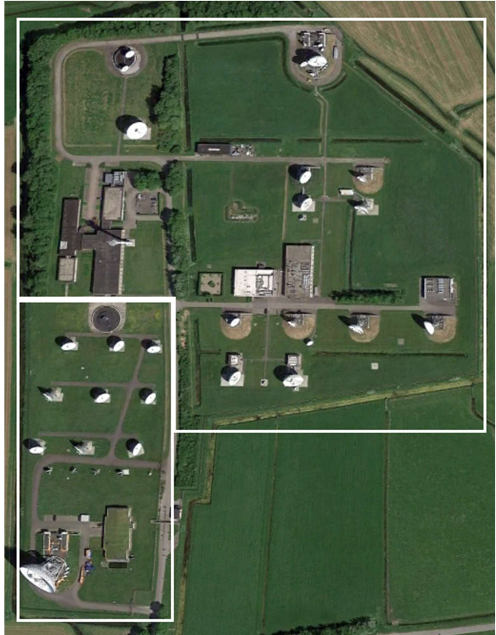
Figure 2.2: Burum SAS (top marked area) and Burum Interception Facility (bottom left marked area).
