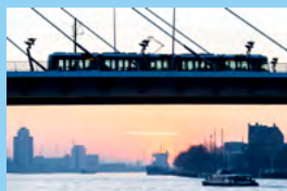
Tram crosses Erasmus Bridge in Rotterdam while water taxi passes below. (p 31)
