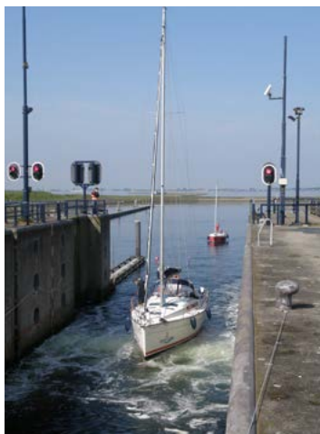
Pilot bellenscherm Krammersluis
