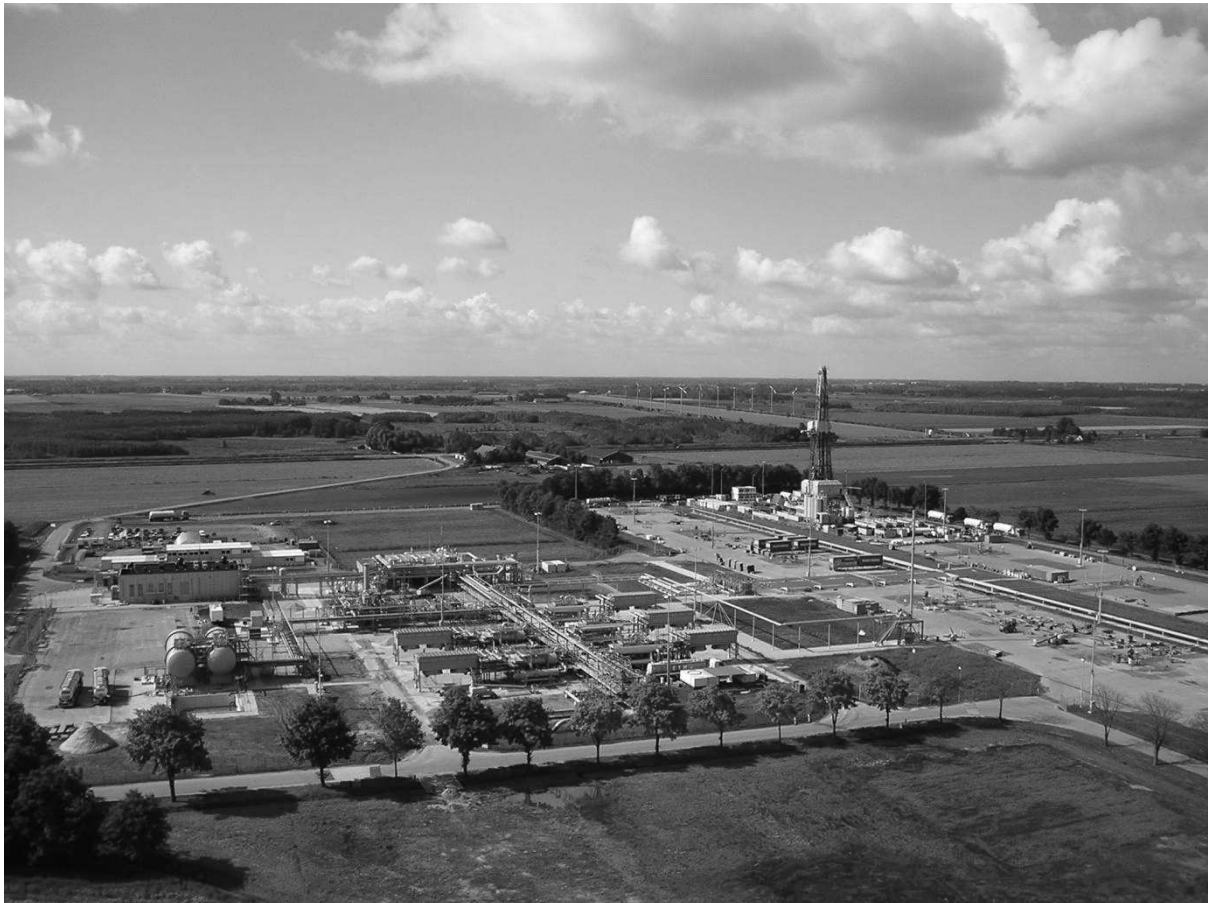
Eemskanaal Cluster with rig drilling Eemsknaal-13
