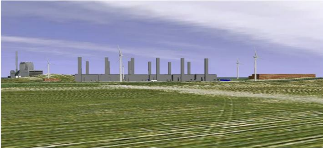
Figure 12.23 ASU plant side view (with existing power plant to the left)
