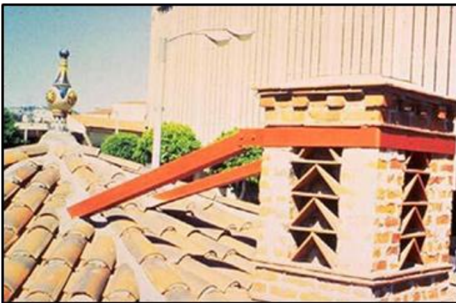
Figure 32 Chimney Restraint
