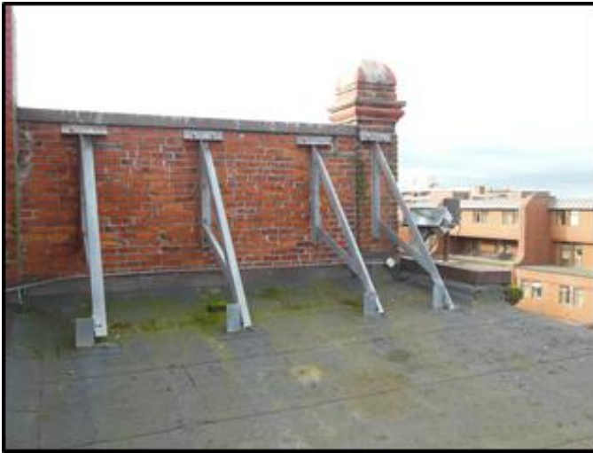
Figure 31 Parapet restraint.
