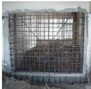
Figure 41 Additional reinforced concrete shear walls
