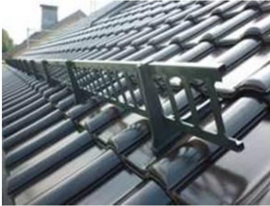
Figure 30 Snow guard rails to capture loose tiles.
