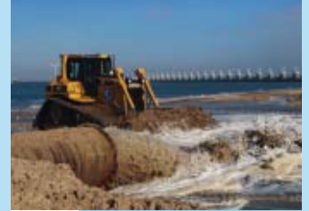
4 Zandsuppletie (sand supplement) (p. 11)
