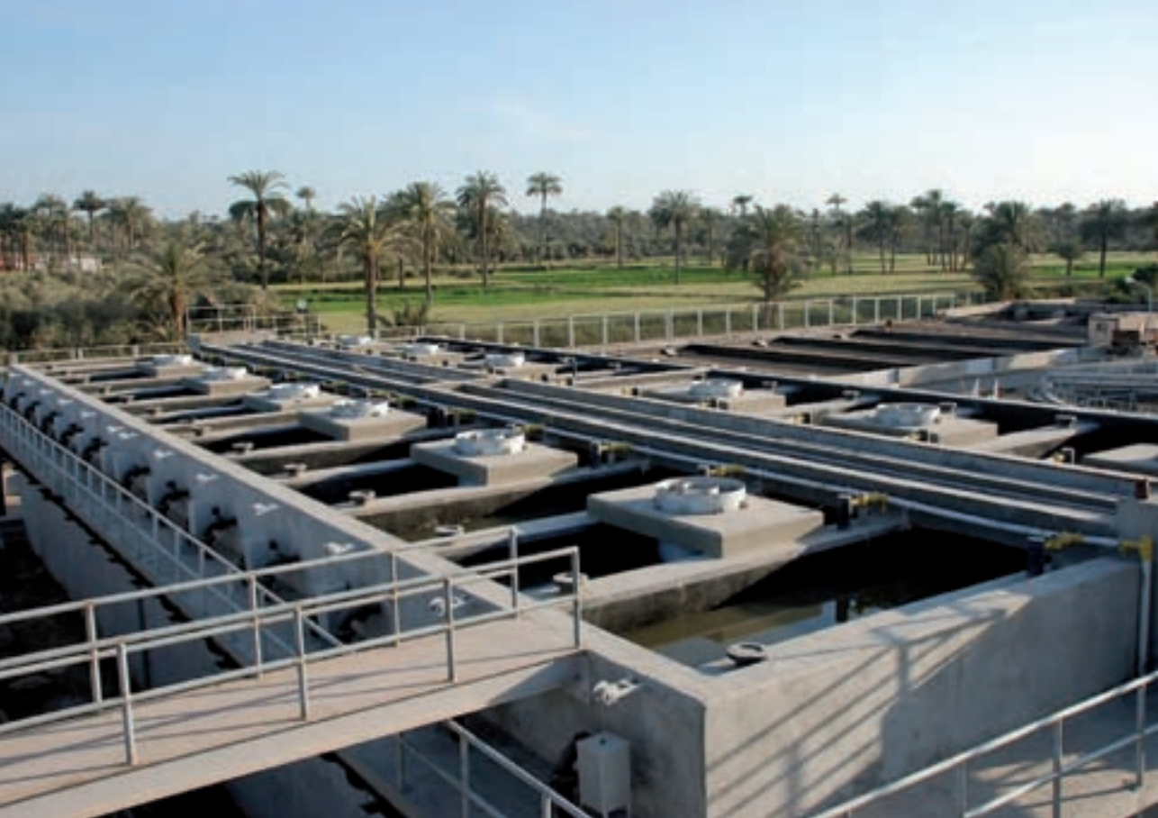
Sanhour UASB Facility
